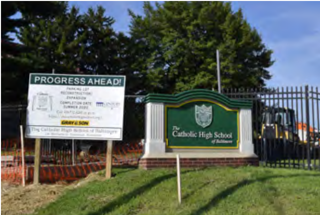
The Parking Lot Project is expected to be completed by October, 2020.
